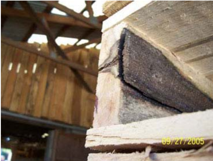
Figure 4f. "Barky" defect in pallet stringer.
